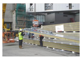
A more typical configuration utilises the double suction pads on traverse extension arms to provide increased panel support and in this form the unit can handle panels weighing up to 1320 lbs.
